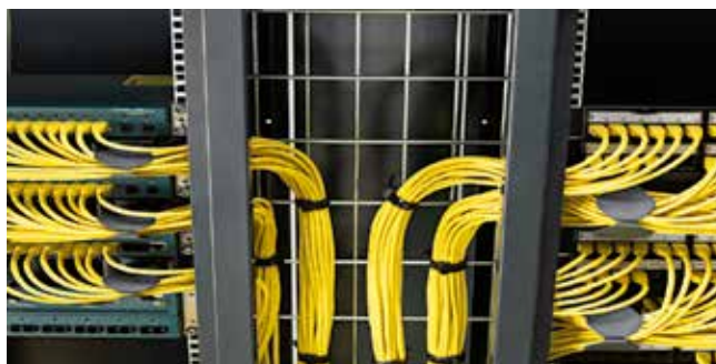
Dedicated space for cable management with easy access via door to cabling unit
